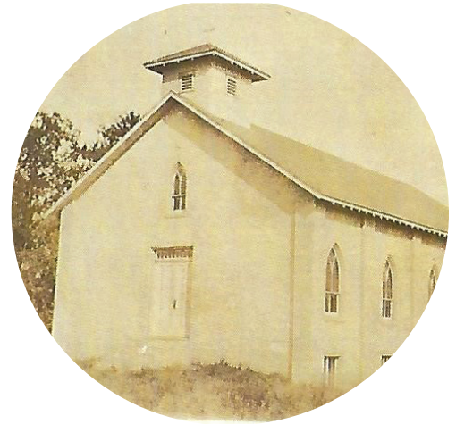
Ascension Catholic Church on Santa Maria Drive was under construction in 1923. Courtesy of Ruth & Bill Rufkahr and CHLPC.
